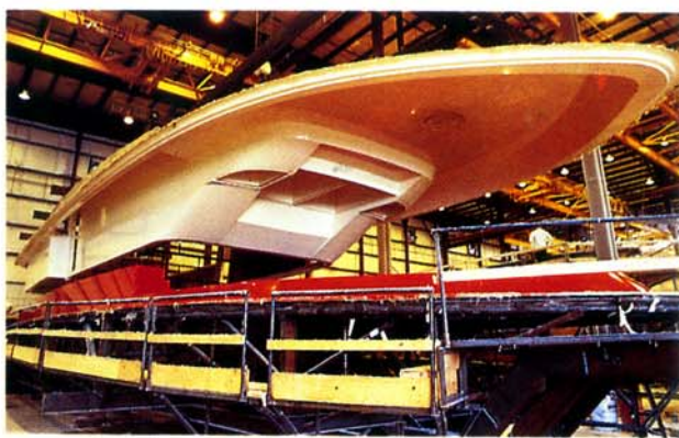
TOPSIDES—The superstructure (here, upside down) uses sandwich materials, tri-axial fabrics.
